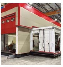
The temporary Station 10 on Hovey Avenue consists of four large fire module apparatus bays that are connected to six trailers that house the kitchen, gym, bunk rooms, bathrooms, and common spaces. The design team, Ted Galante Architecture Studio, presented the City with this creative solution of building a modular fire station to house equipment and staff during the renovation.
